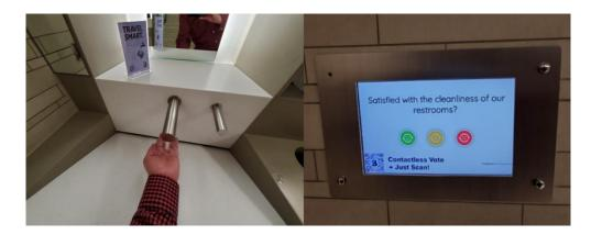
Figure 4.5 Contactless faucet and feedback systems for cleanliness in restrooms.
